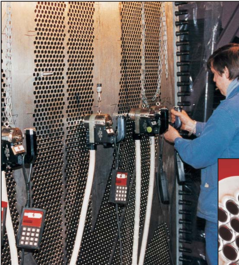
Shown welding titanium heat exchangers
