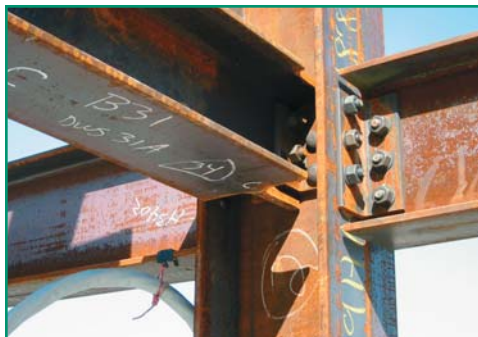
Beam connections are fast and economical – meeting your toughest construction deadlines.
